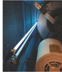
UV-C light keeps coils free of mold
