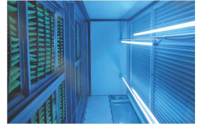
UV-C light keeps coils free of mold
