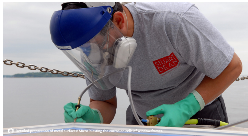
📷 Detailed preparation of metal surfaces: Micro-blasting the corrosion cells of window frames.
