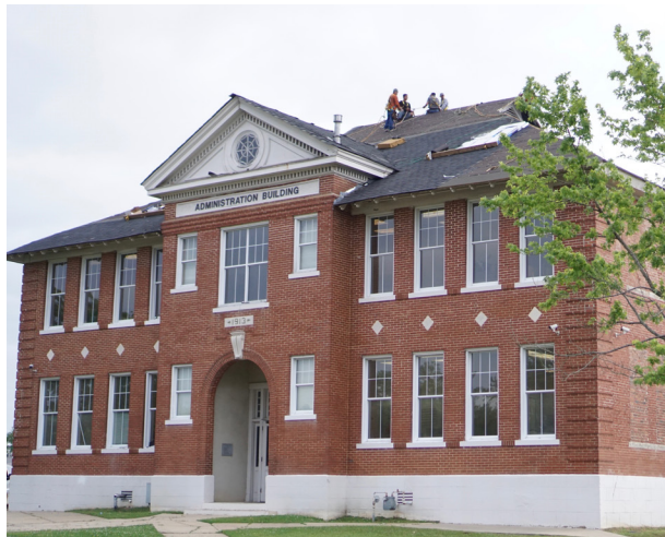
Sheridan School District’s Admin Building, built in 1913, still operational today, and required special attention during district-wide roofing project
