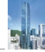
One Island East Hong Kong, China BEAM Platinum
