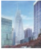
Bank of America / One Bryant Park New York, USA LEED Platinum
